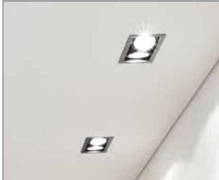
Retro Fit in Hallway
