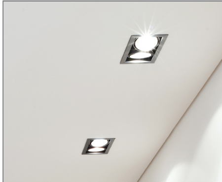
Retro Fit in Hallway
